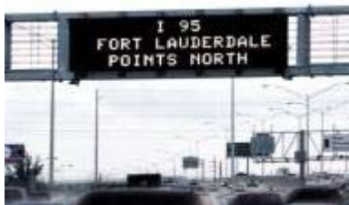
Fig 3. Existing Overhead Sign Converted to NTCIP.
