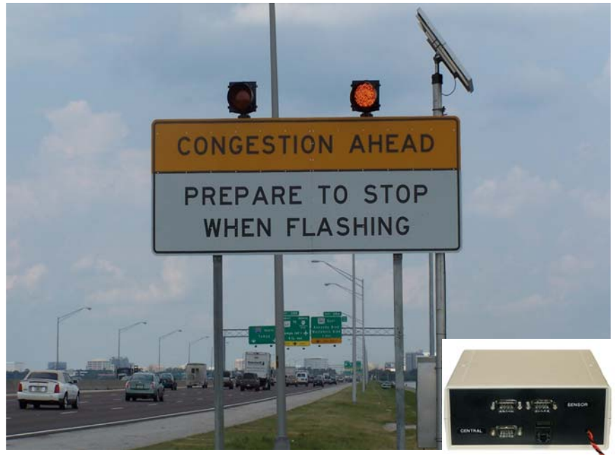
Fig 4. Warning Drivers of a Collision Danger Ahead in Tampa. Inset: IDI2500 Traffic Congestion Monitor
